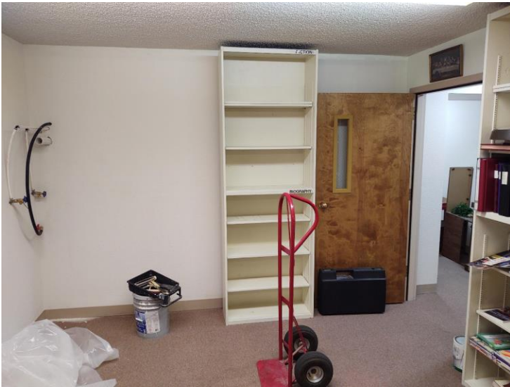
East Wall Showing New Water/Drain and Gas Utilities
