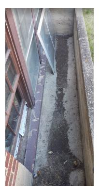
**Grout** – Grout the seams (left and right) of the window wells on the west side of the church as the cement has pulled away from the foundation leaving a void for water to flow in from the grassy impoundment that can get overwhelmed by the volume of water coming off the roof.
