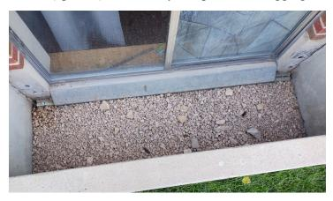
Center Window Well - Remove French Drain/Concrete Floor – Currently the floor of the center windows well is cemented with a French drain. We propose demoing out the cement, digging down about 4' then filling the void with rock aggregate.
